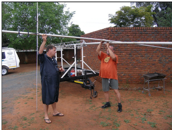
Hans ZR6HVG and Pieter ZS6PA erecting portable 6m and 2m yagis as well as a 1.3 GHz helical
